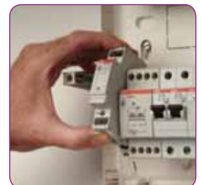
DIN RAIL MOUNTED COMPONENTS Bell Transformers, timers, contactors etc.
